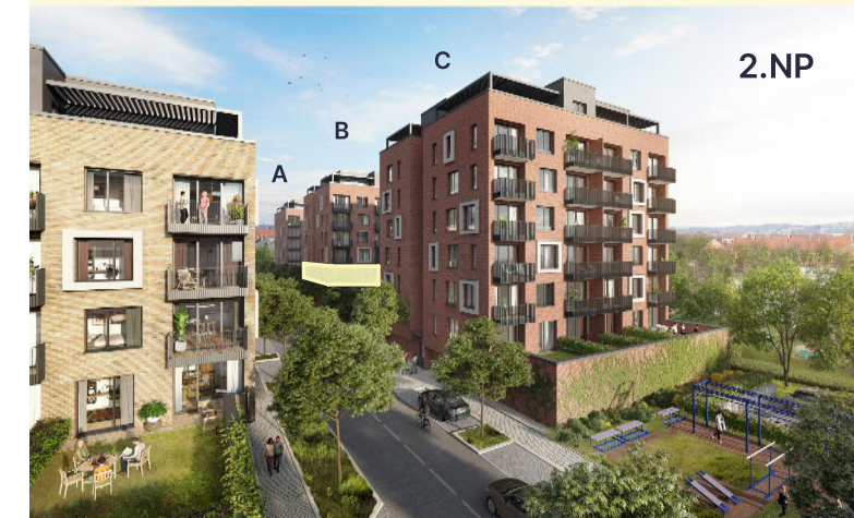
Pohled na dům / Building View
