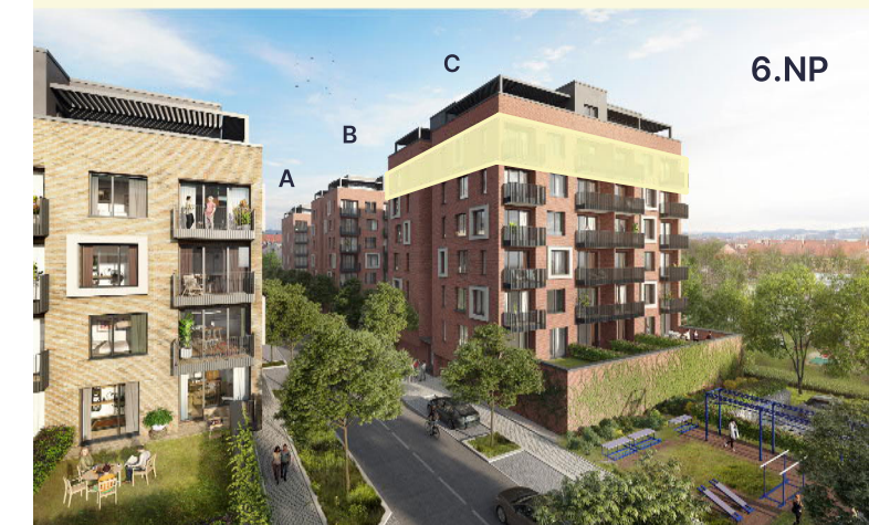
Pohled na dům / Building View
